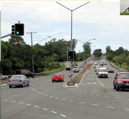
Morayfield Road, Centenary Lakes after the recent flood
