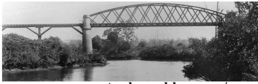
www.moretonbay.qld.gov.au/ Caboolture River & Rail Bridge
